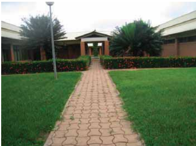
Photo 3. Main entrance of Building A
