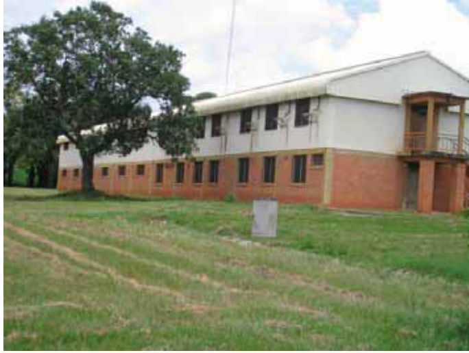
Photo 7. Building F (Administration and Finance)
