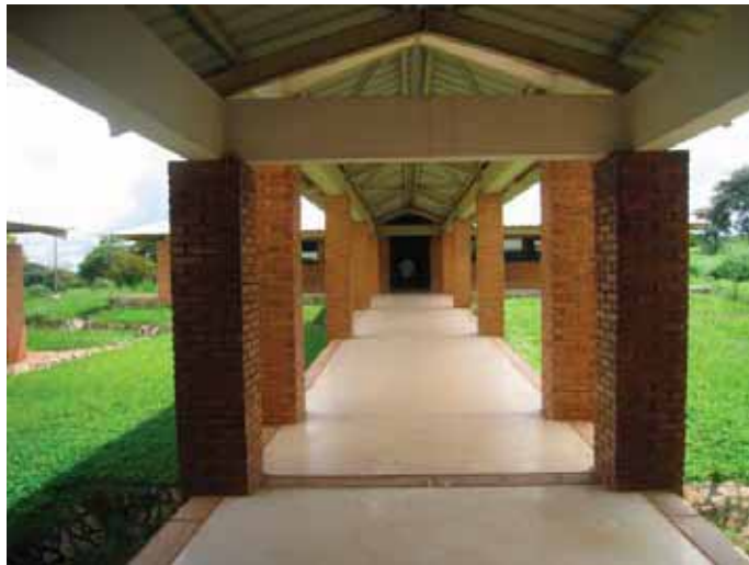
Photo 6. Main entrance of building B
